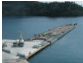
Ferry Pier L143m x B20m x D3m
