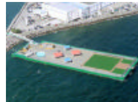
Shimizu Port Fishing Park L143m x B20m x D3m
