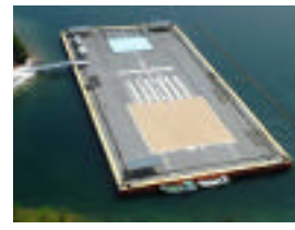
Marine Park Kumanonada L120m x B60m x D3m
