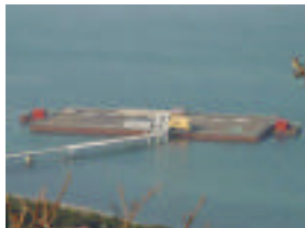
Uzushio Megafloat Nandan L101m x B60m x D3m
